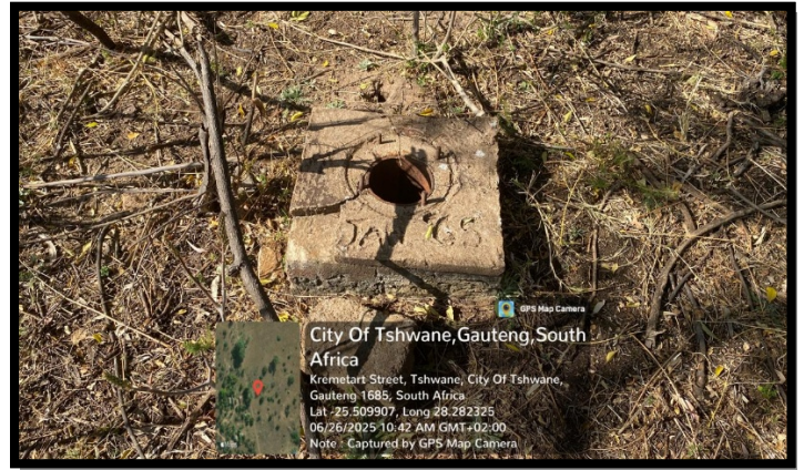
Figure 10: Old Borehole Structure
